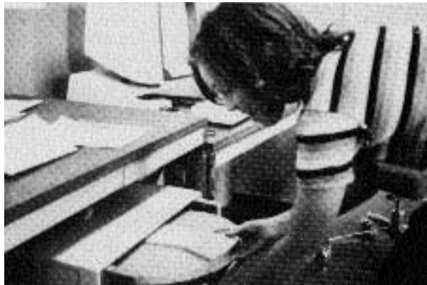
Figure 26.4. Inserting the disk pack in the Dynabook.
